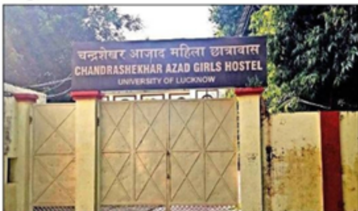
SET FOR RENOVATION: Chandra Shekhar Azad Girls' Hostel
