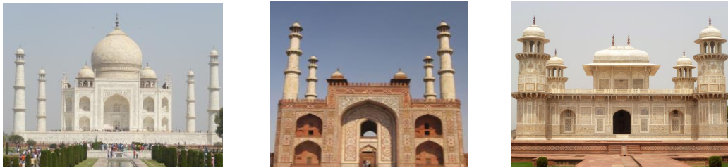
Figure 36 Symmetry in Structures of Mughal Buildings in Agra
