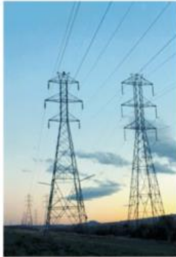
Figure 3: High Voltage Transmission Line
